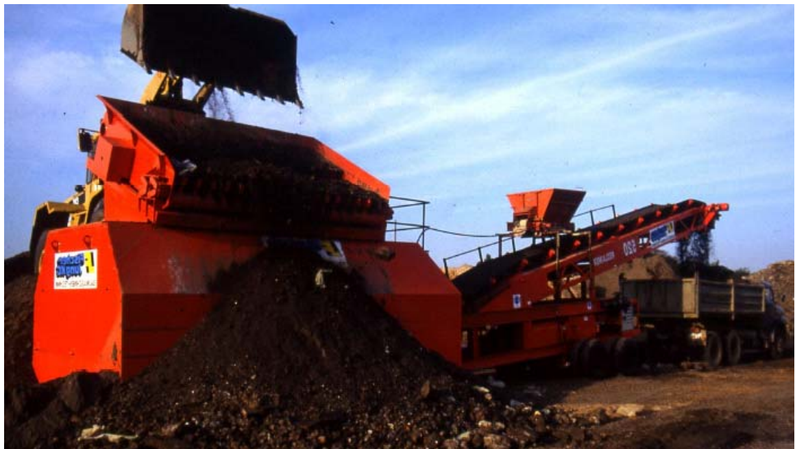
Figure 5-24: Bulking of contaminated soil
