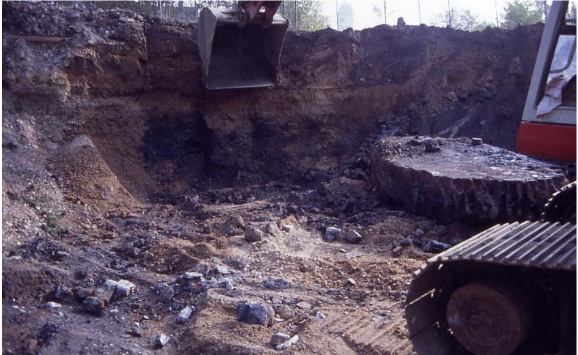
Figure 5-23: Excavation of contaminated soil
