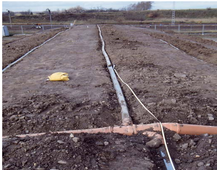
Figure 5-31: Internals for Water Management and Aeration of Windrows [Institute for Microbiology, Braunschweig/Germany]
