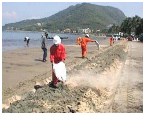
Figure 5-22: Addition of nutrients to a contaminated beach [VIT, 2003]
