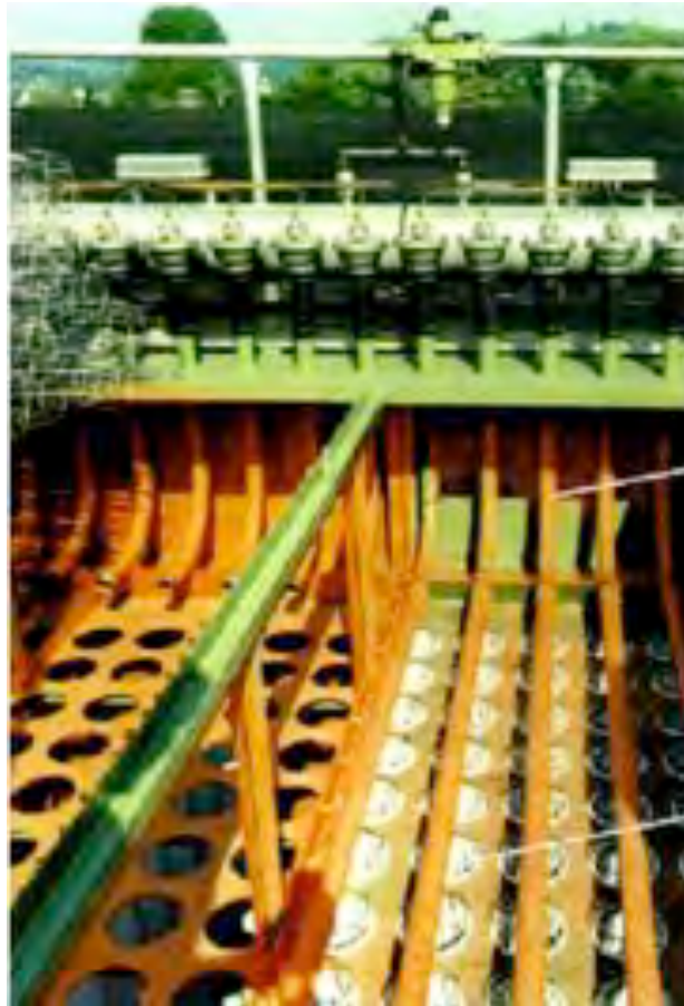
Figure 5.4-10: Fabric filter [Igelbüscher, 2005]
