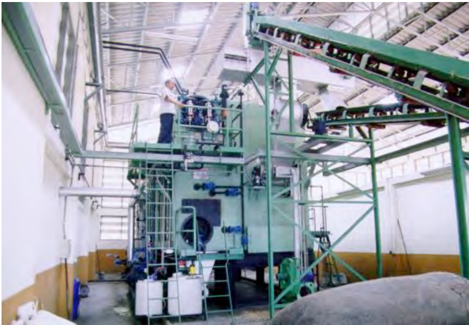
Figure 9.3-1: Fluidized bed boiler for superheated steam production of 5 tonnes/hr at 30 barg, 350°C
