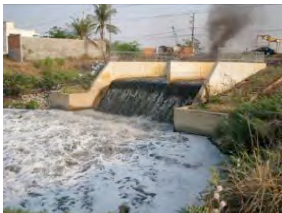
Figure 3.2-1: Discharge site of sewage system in Phnom Penh
