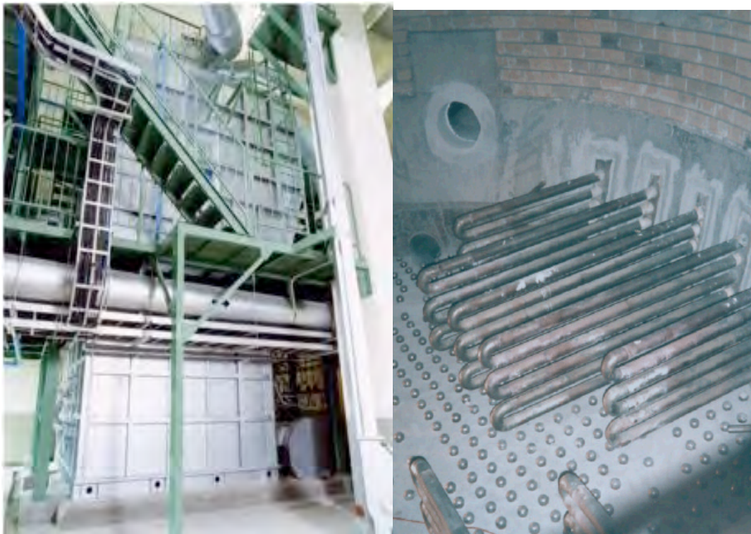
Figure 5.4-7 (left): Fluidized-bed reactor
